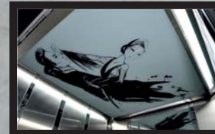
Armatürde kullanılan dijital baskılı cam ve yanlarda led aydınlatma UV printed glass and side LED lighting on ceiling
